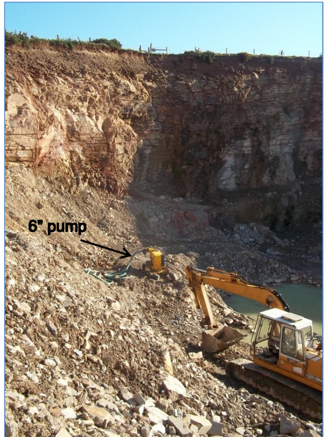
Plate PP/10: View of eastern face (30/09/2011) with extraction currently underway at base of quarry. Excavator fitted with bucket.
