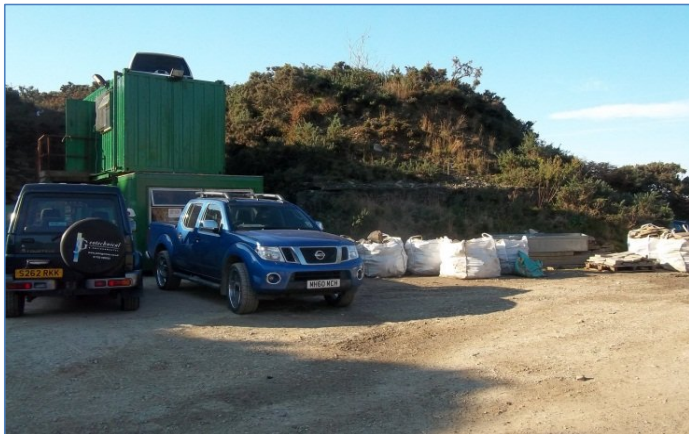
Plate 2: Site offices and compound in 2011.
