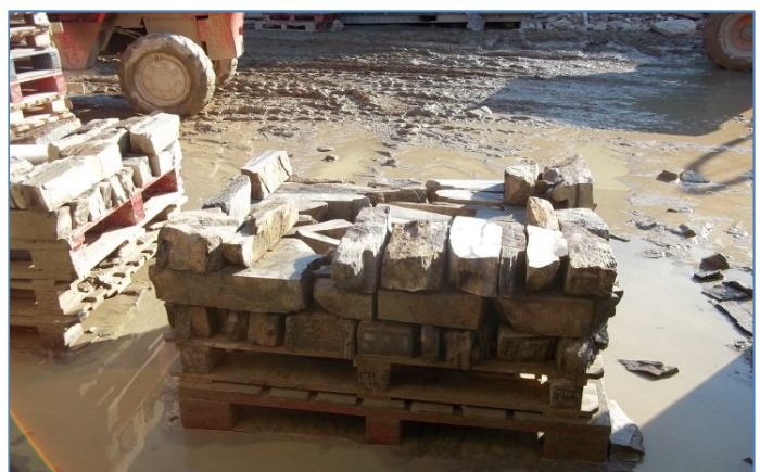
Plate PP/8: Cut stone loaded by hand onto pallets.
